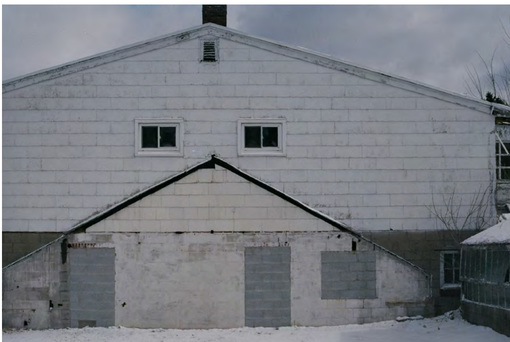
Figure 3-5: The main house – Used with permission 101
